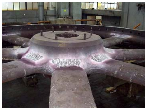
Large cracks found in spider of hydrogenerator. Figure 6.
